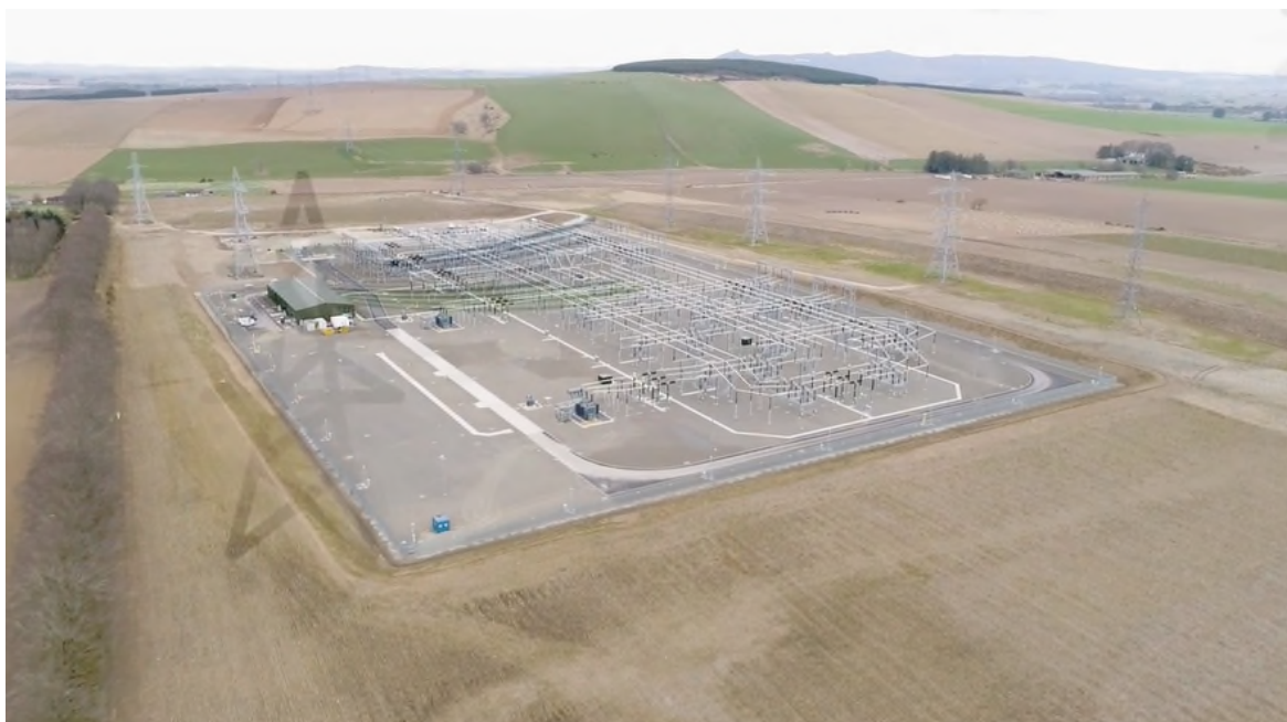
Photo 1: Looking south across Rothienorman sub-station site. Subject site to east of this.
